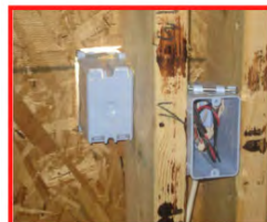
Electrical box not air sealed.
