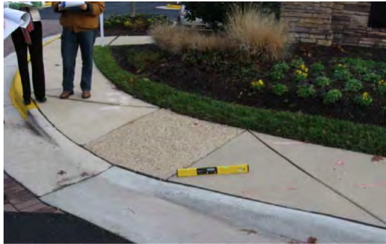
Common Compliance Oversight: Curb Ramp Creates Excessive Cross Slope
